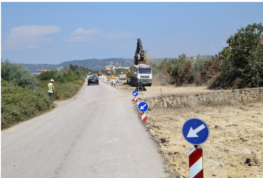
(18) The widening of more than double width of the road which connects the airport with the highway
