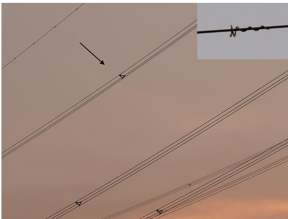
Figure 6. High voltage (380 kV) transmission line with spacers (arrow) to keep individual energised phase conductors in each bundle apart. The single thin wire in the top left corner of the photo is the ground wire (also called neutral or earth wire) that is mostly positioned above the phase conductors. In this case the ground wire has been equipped with small spirals (so called pig tails, see inset) to make this wire better visible to birds (Photo: Bureau Waardenburg).
