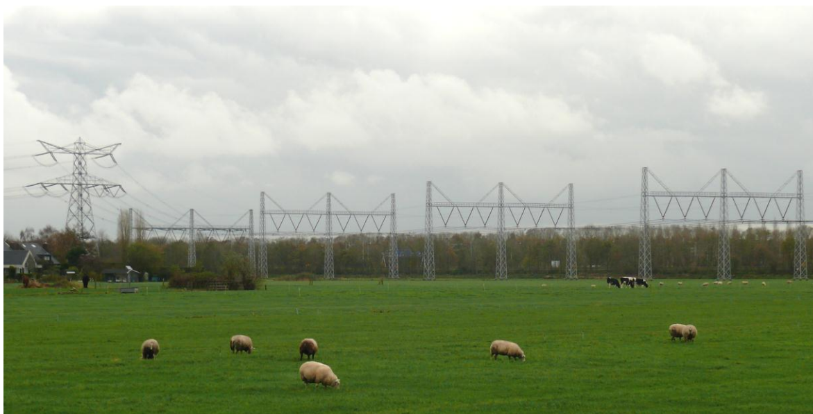
Figure 7. A 380 kV line, with lowered conductor wires hanging from portals in one horizontal plane to minimise collision risk for Great Cormorant ( Phalacrocorax carbo ), Eurasian Spoonbill ( Platalea leucorodia ) and Purple Heron ( Ardea purpurea ) daily passing this stretch of line while commuting between the breeding colony and foraging areas, Muiden, the Netherlands (Photo: Bureau Waardenburg).
