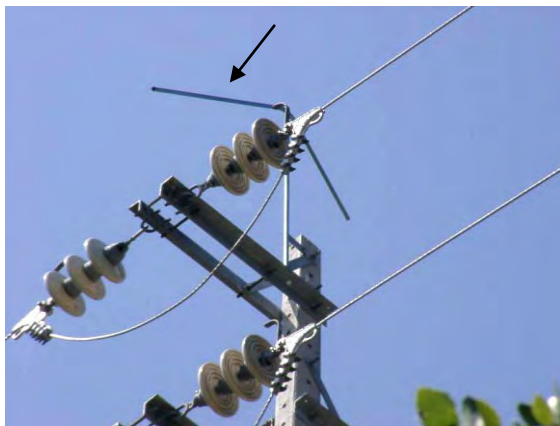
Figure 11. Distribution pole with symmetric chevron (arrow) on top as bird exclusion device (Photo: EDP-Distribution, Portugal; and distribution pole with bird exclusion spikes with dedicated nesting pole for White Stork next to it (Photo: Carlos Tiago).
