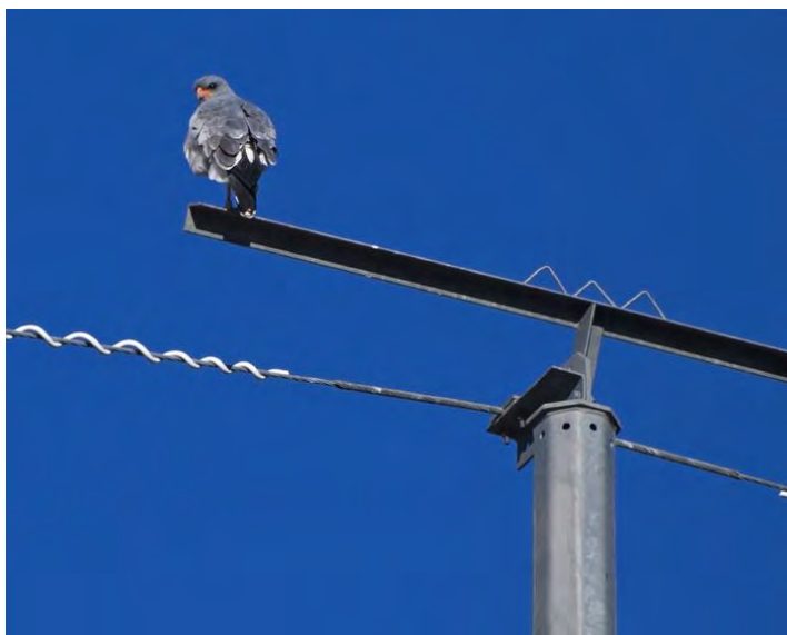
Figure 11. Distribution pole with symmetric chevron (arrow) on top as bird exclusion device (Photo: EDP-Distribution, Portugal; and distribution pole with bird exclusion spikes with dedicated nesting pole for White Stork next to it (Photo: Carlos Tiago).
