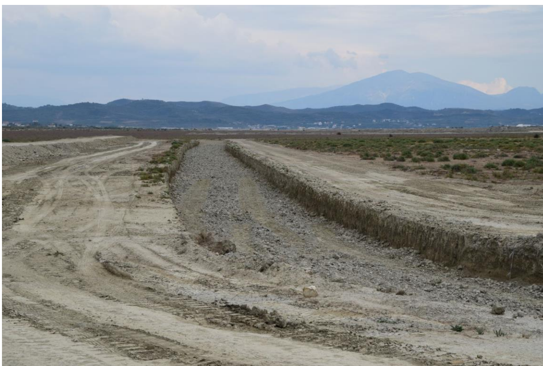
(17) The perimetric drainage ditch of the airport
