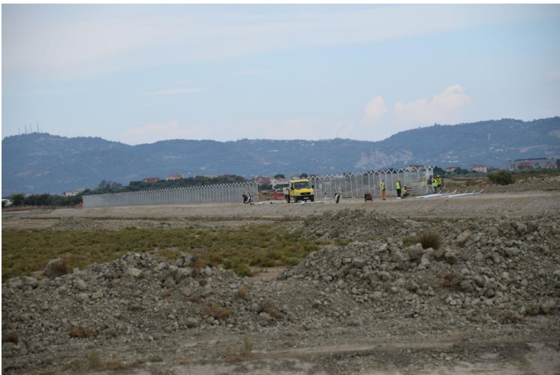
(13) The starting of the fence construction
