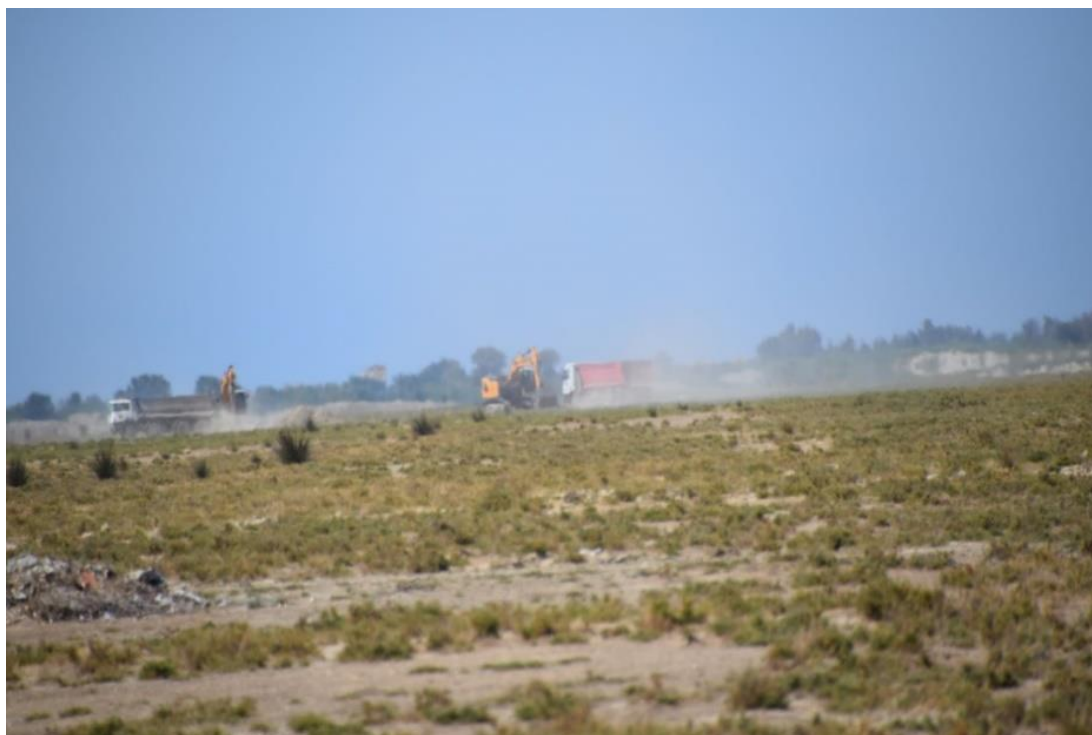
(16) Soil excavation tasks in progress
