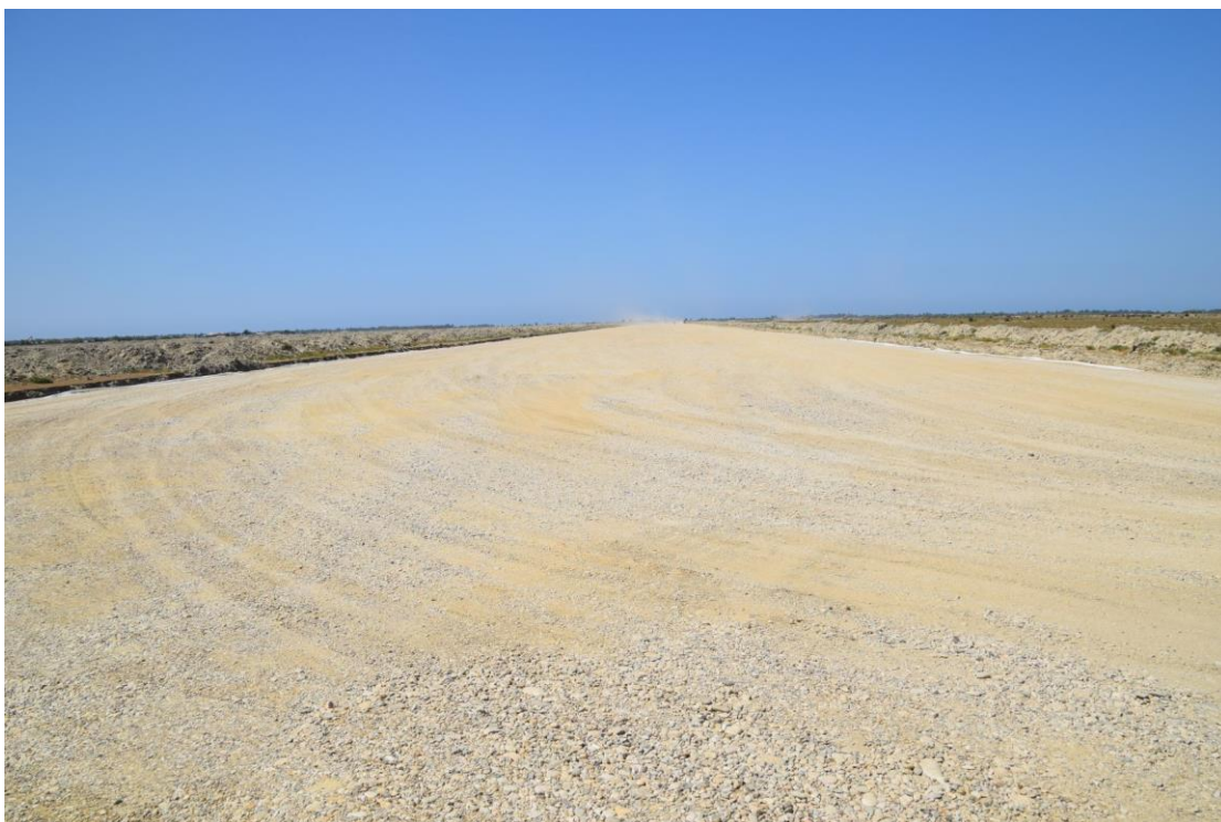
(14) The runway of the airport from the east side
